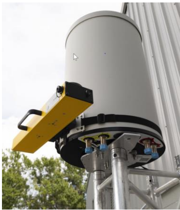
Small Cell Mount on Antenna (with and without AAT)
